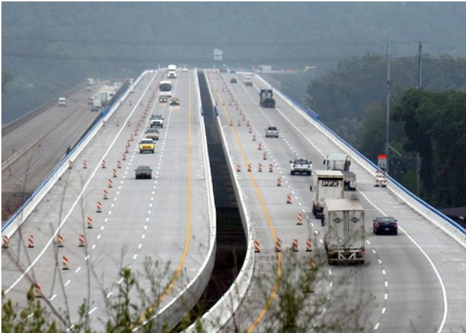
HT Rail (TL5) Susquehanna River Bridge Harrisburg, Pennsylvania
