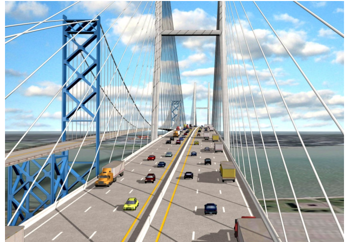
Gordie Howe International Bridge (Windsor-Detroit) Detroit and Ontario, Opening 2020
