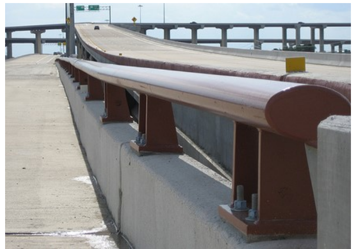
TxDOT T4 Painted TL-3 (42" tall) SH 620 at US 183, Austin, Texas
