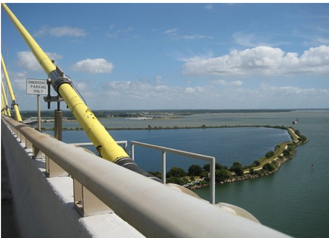
TxDOT T4 TL-3 Fred Hartman Bridge, Baytown, Texas
