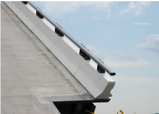
TH80 (TL5) on I-95 over Potomac River Woodrow Wilson Memorial Bridge, Maryland
