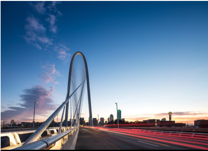
TxDOT HT TL-5, Designed by Santiago Calatrava Margaret Hunt Hill Bridge, Dallas, Texas
