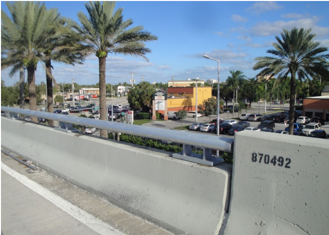
FDOT T401 (TxDOT Standard) SH 94, Miami, Florida
