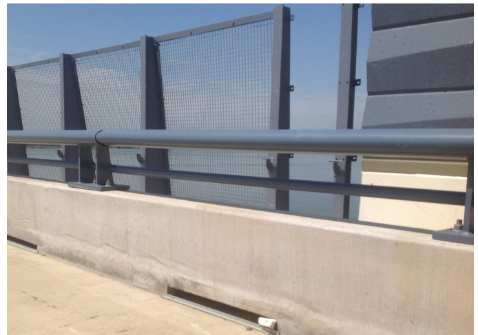
TxDOT C402 Painted TL-3 Lake Lewisville Bridge, Lewisville, Texas
